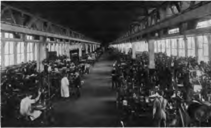
Fig. 1. Individual Motor Drives.
